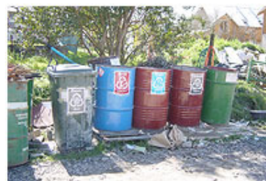
Sorting bins for the builders on-site
